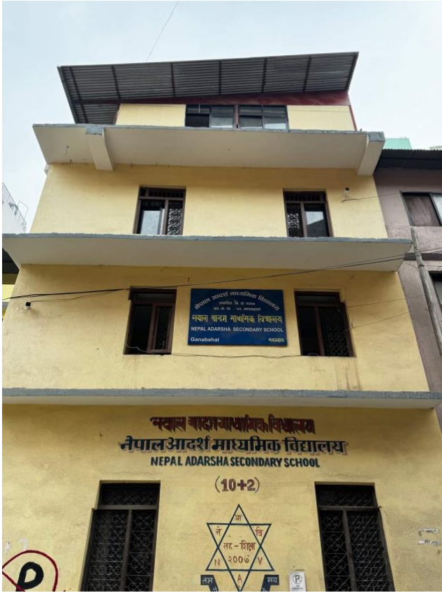
Newly completed school buildings at Nepal Adarsha School (left). The school operates from two buildings separated by a relatively busy road.
