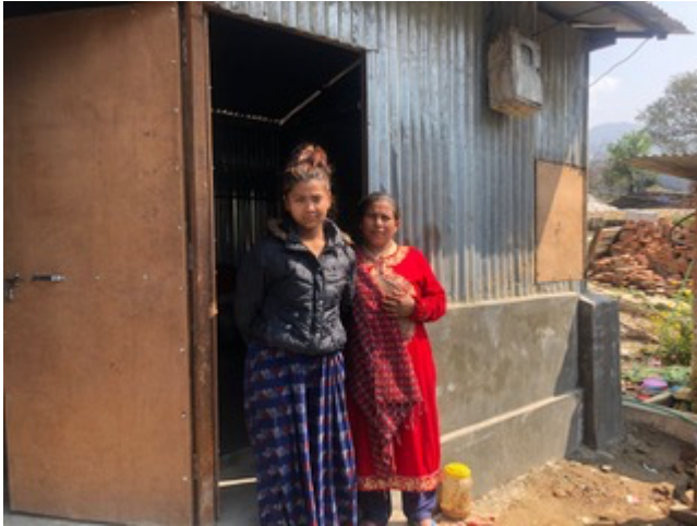
Left shows the zinc house when completed early 2022 – Nita with her mother.
